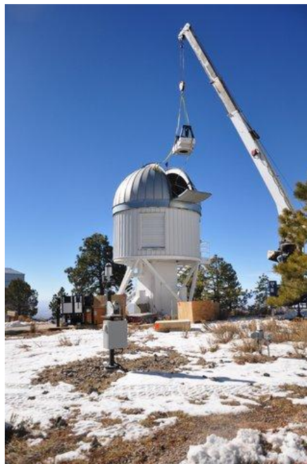
The telescope at APO – a 1m Alt/Az PlaneWave CDK1000 telescope system – was installed on the 17th of January 2024. Credit: Jason Jackiewicz
