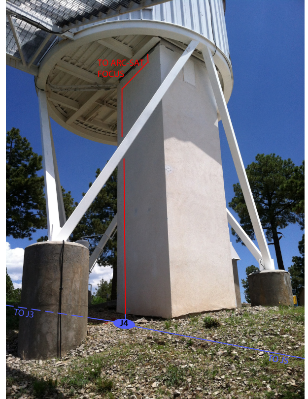
FIG. 5.— Junction box 4 (J4) shown with the underground runs to J3 and J5 in blue. The single conduit run for the PT can be seen in red coming up the pier of J4 to the observing level of the ARCSAT telescope.
