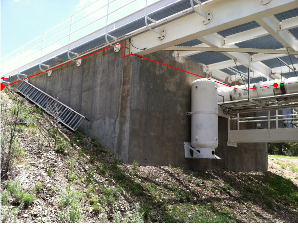
FIG. 6.— Above ground cable tray from just after J5 to the junction with the existing APOGEE fiber run tray under the 2.5 m mechanical level. The J5 box is just off the image to the left. The red line indicates the intended run of new cable tray. The red dot is the intersection with the existing APOGEE cable tray and finally the green line indicates the continuation of the existing APOGEE fiber run. Dashed lines indicated the cable tray is behind something in the image.
