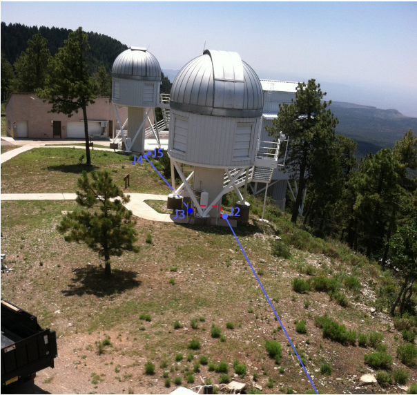
FIG. 2.— The full underground run is shown in blue as seen from the observing level of the 3.5 m telescope. In order from the foreground are the NMSU 1 m, ARCSAT, and the SDSS telescope. The brown building in the far ground is the SDSS plug lab and the APOGEE spectrograph room where the existing fiber run terminates. Dashed lines indicate the fiber run is passing behind something in the image..
