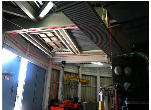
FIG. 3.— Image of the lower level of the 3.5 m telescope enclosure with fiber roughing marked. The green line represents existing cable trays. The red line is the proposed routing for the new cable tray. The new cable tray stays clear of both the 3.5 m primary mirror hatches and the loading dock doors. A red dot on the wall at the far side of the door indicates the wall pass trough to J1. Dashed lines indicate the conduit is routed behind something in the image.
