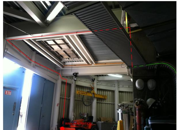
FIG. 3.— Image of the lower level of the 3.5 m telescope enclosure with fiber routing marked. The green line represents existing cable trays. The red line is the proposed routing for the new cable tray. The new cable tray stays clear of both the 3.5 m primary mirror hatches and the loading dock doors. A red dot on the wall at the far side of the door indicates the wall pass through to J1. Dashed lines indicate the conduit is routed behind something in the image.
